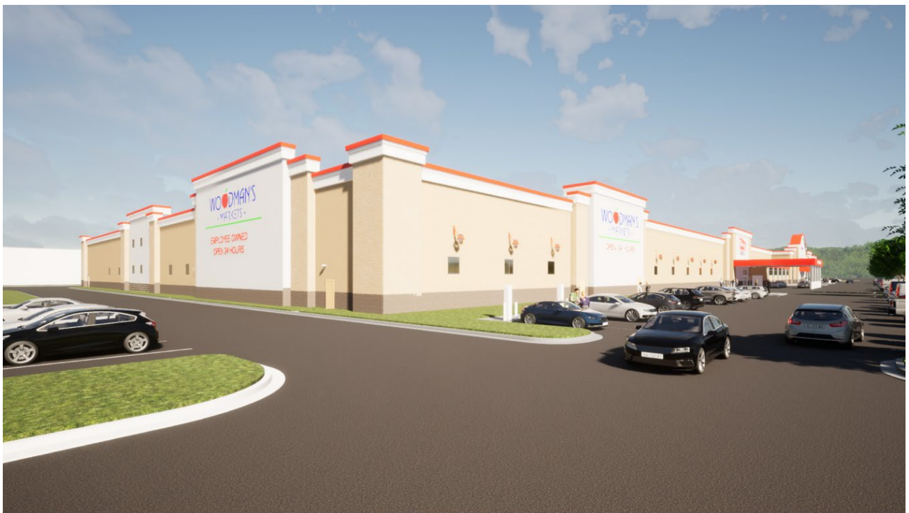
Woodman's Food Market West/South Façade (Looking Northeast)
