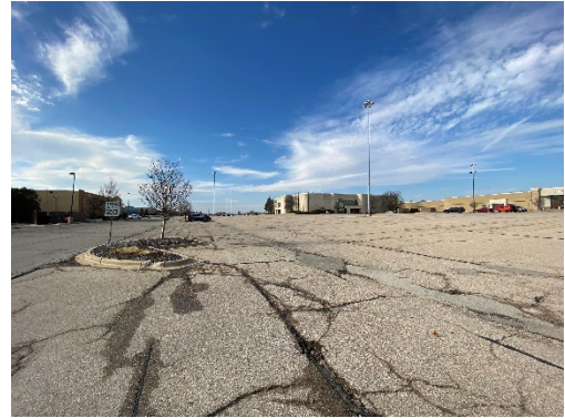
Looking East at alley/neighbor
