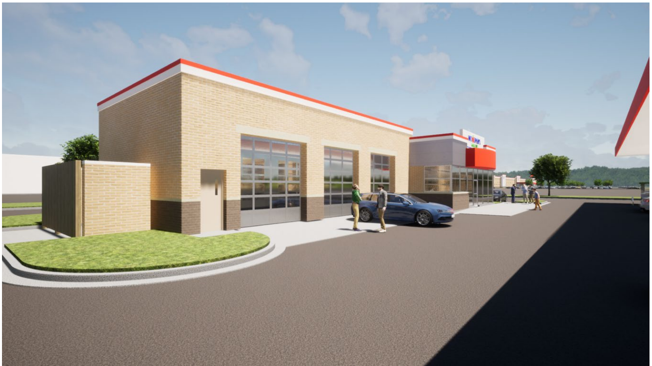
Woodman's Gas Station South Façade (Looking Northeast)
