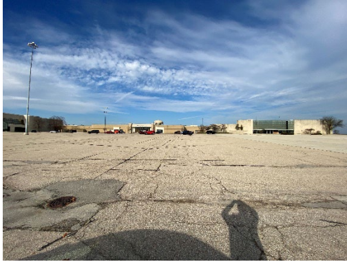
Looking West at alley/neighbor
