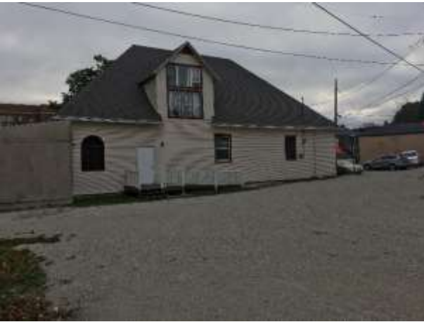
Looking north at the existing structure from St. Patrick Street
