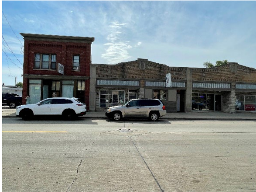
Looking east at subject property
