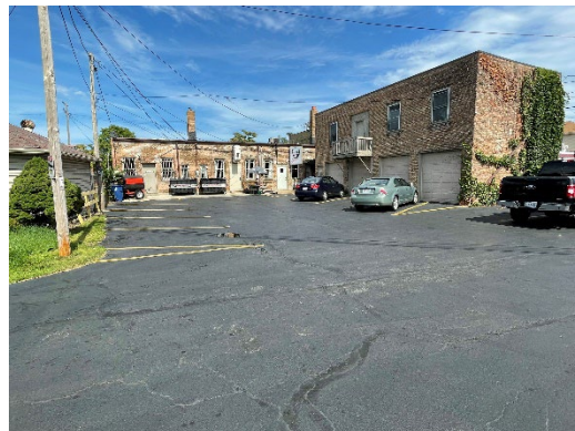
Looking at the rear of subject property
