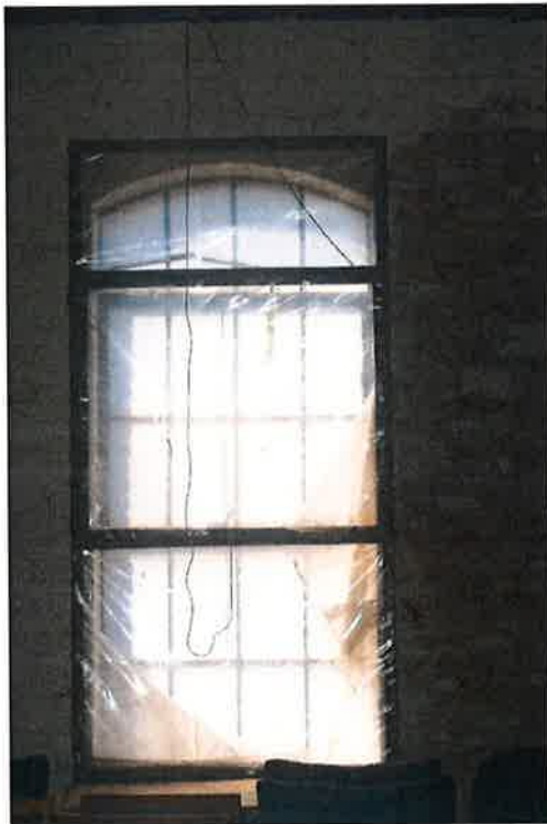
554 / INTERIOR (EXTERIOR NOT ACCESSIBLE)
