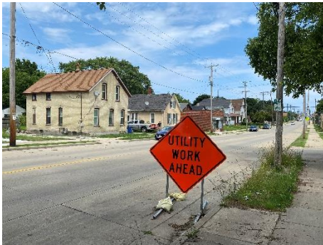
Looking Northeast down High Street
