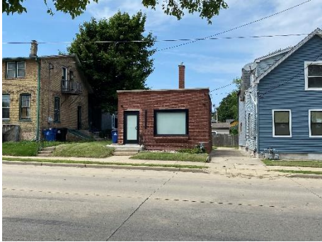
Looking North at the structure
