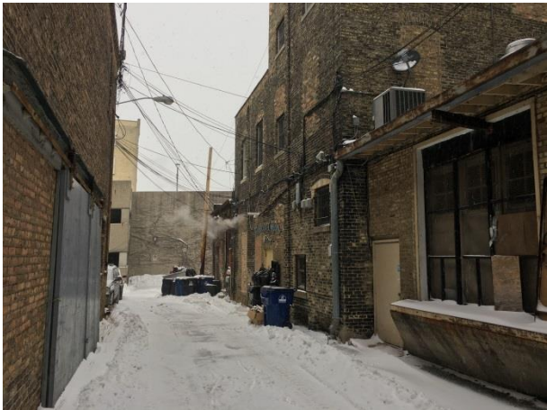
Close up of rear of subject property
