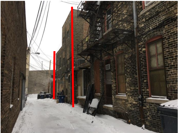
Looking at rear of subject property (red)
