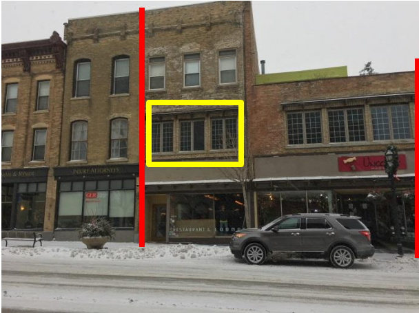
Looking (west) at subject property (red) tenant space shown in yellow
