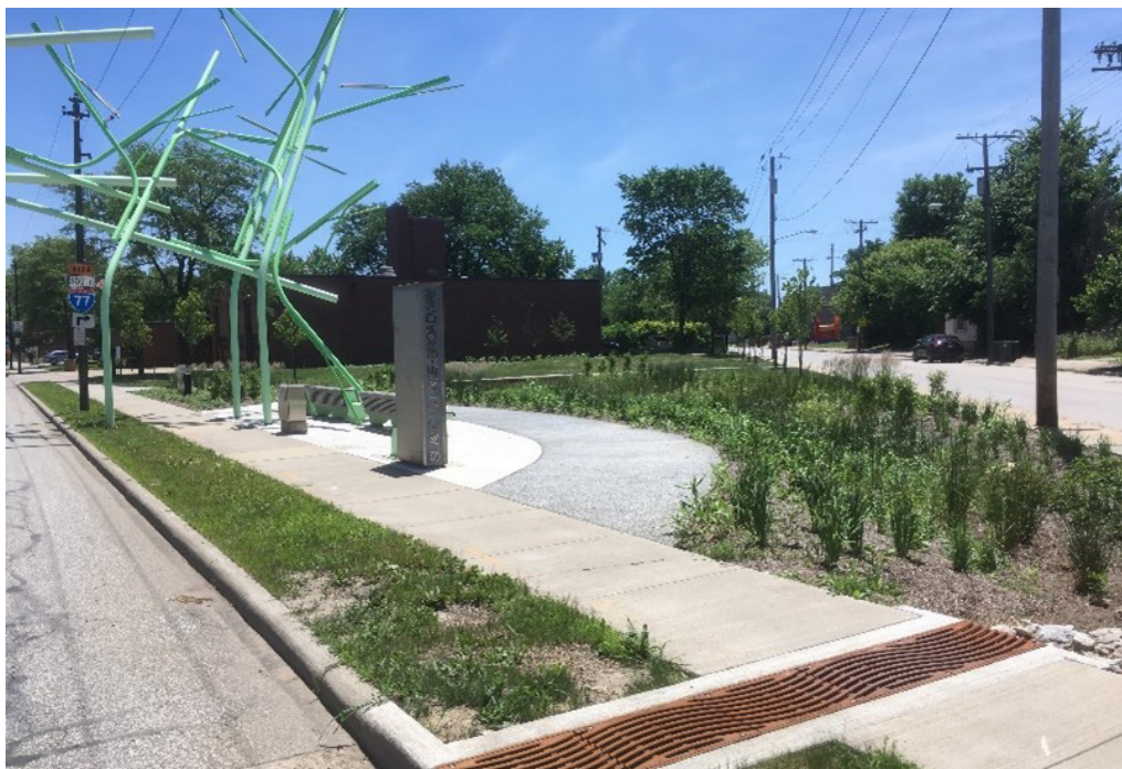
Arch Park Green Infrastructure Park, Cleveland, Ohio
