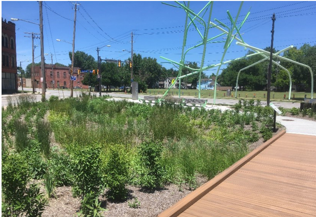
Arch Park Green Infrastructure Park, Cleveland, Ohio
