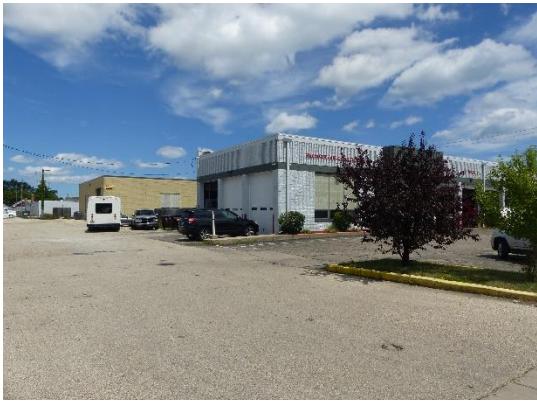
North East at existing building
