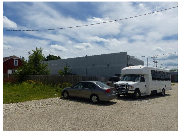
Looking South East at rear of building (where addition will go)
