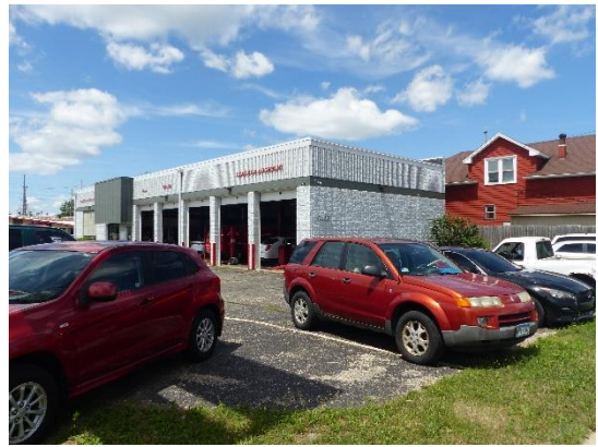
Looking North West at existing building
