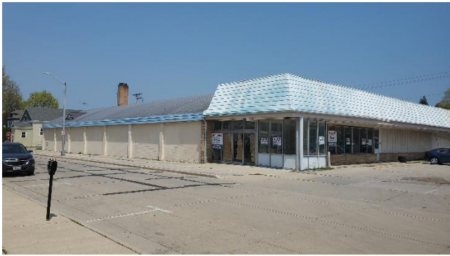
Looking Northeast at site
