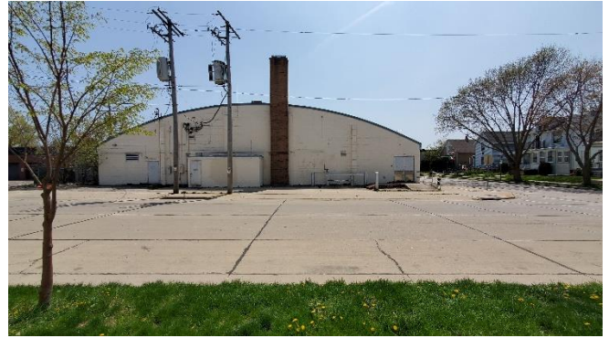
Looking south at the building
