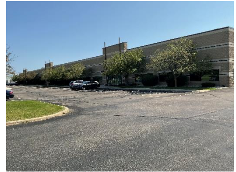
Looking northeast at site (Memorial Drive)
