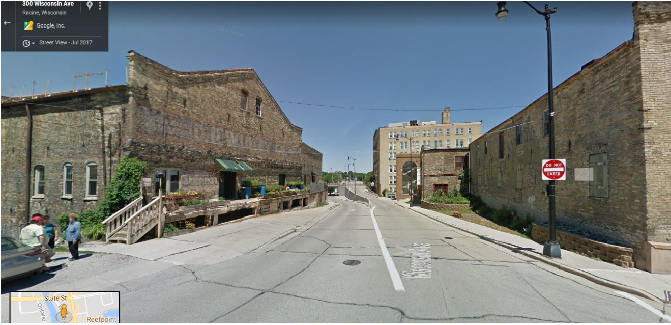
Looking north on Wisconsin Avenue.
