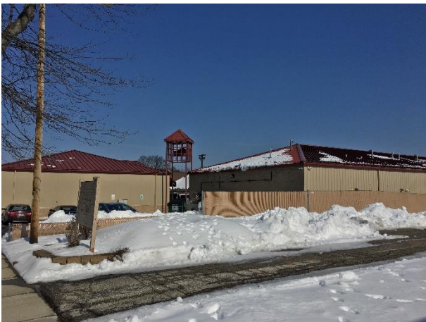
Looking north at the rear of the shopping center from the southern lot line
