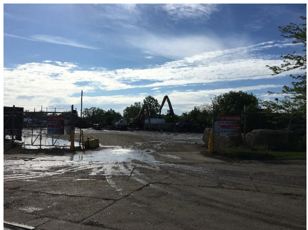
Looking east at subject property from Holborn Street.
