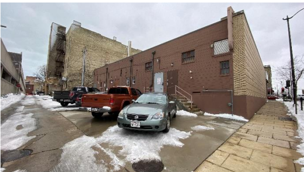
Looking at east side of building (rear)
