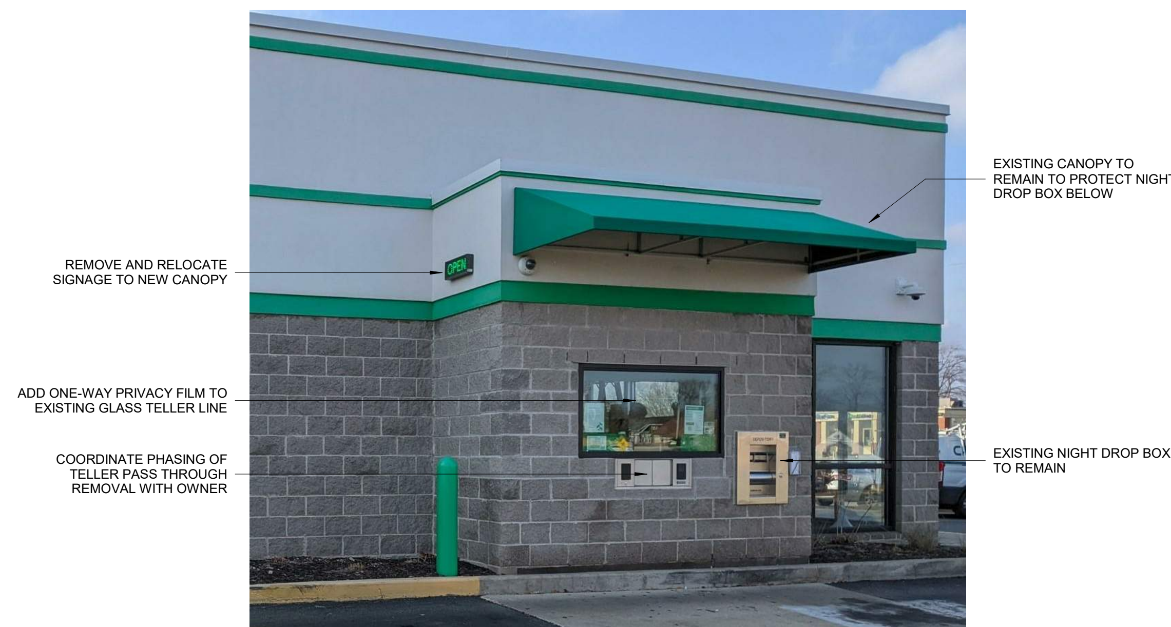
4 EXISTING BUILDING DRIVE THRU WINDOW 3/8" = 1'-0"
