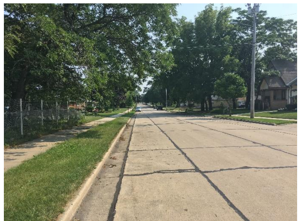
Looking south along Russet Street
