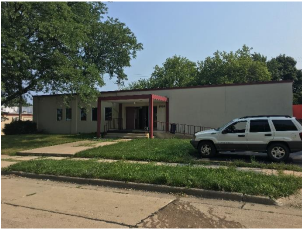
Looking south at the subject property
