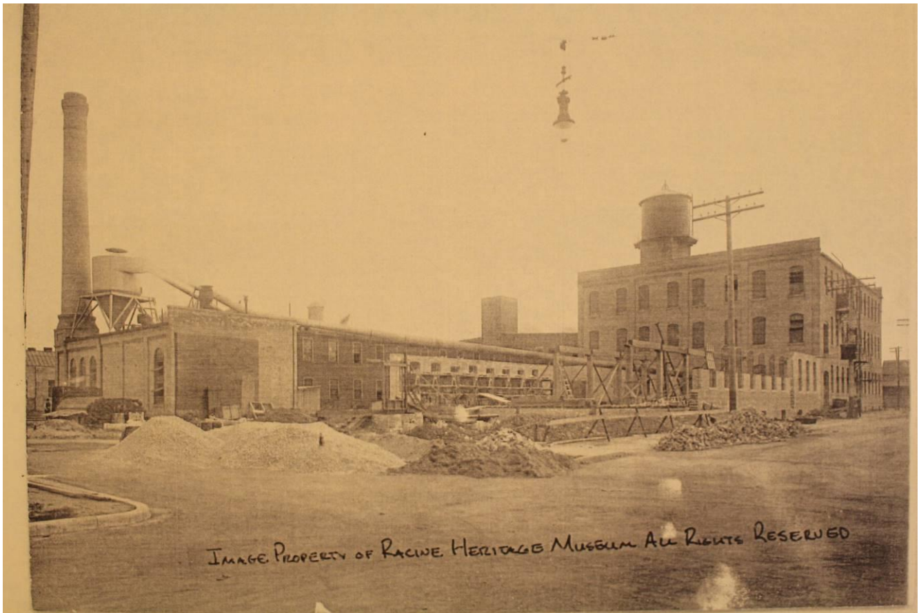
Figure 11: View of c.1917 addition under construction – looking southwest. Racine Heritage Museum
