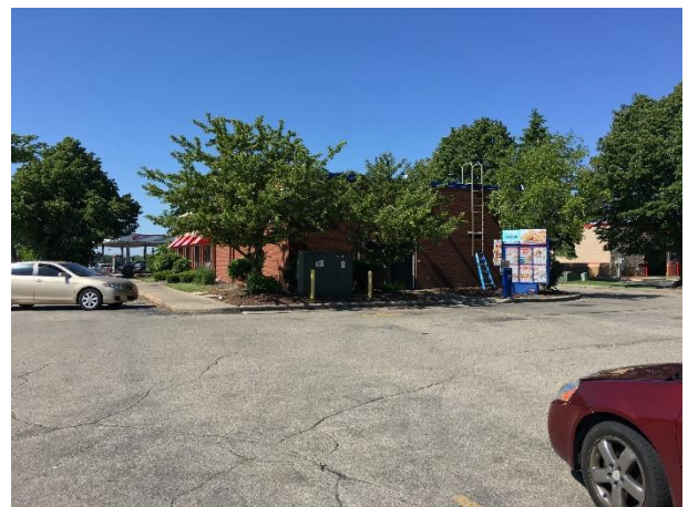
Looking south at rear of building from subject property
