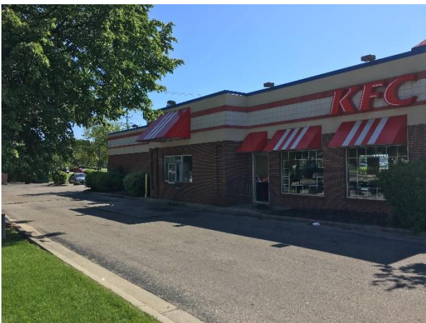
Looking at west side of building from subject property
