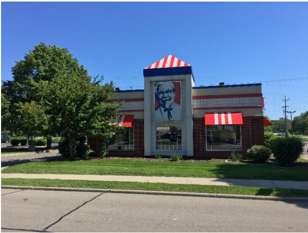
Looking north from 21 st Street at subject property
