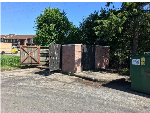
Looking at existing trash enclosure at rear of property
