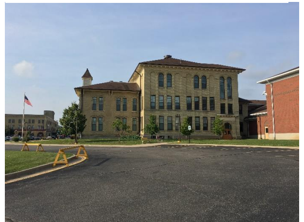
Looking at north elevation of school building
