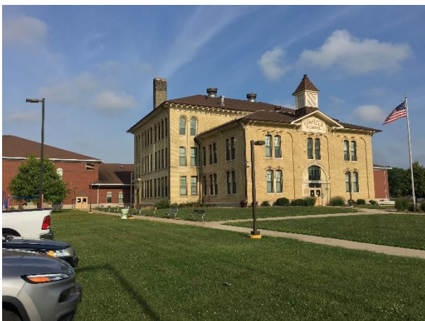
Looking at south and east elevation of building
