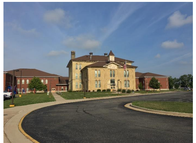
Looking at east elevation of building
