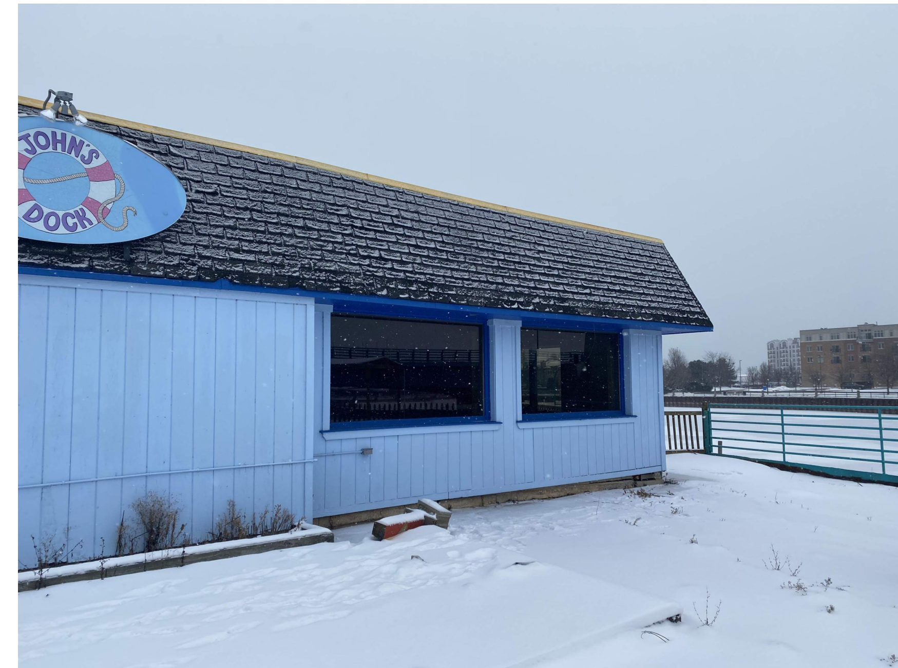
EXISTING BUILDING SIDE (WEST) FACE
