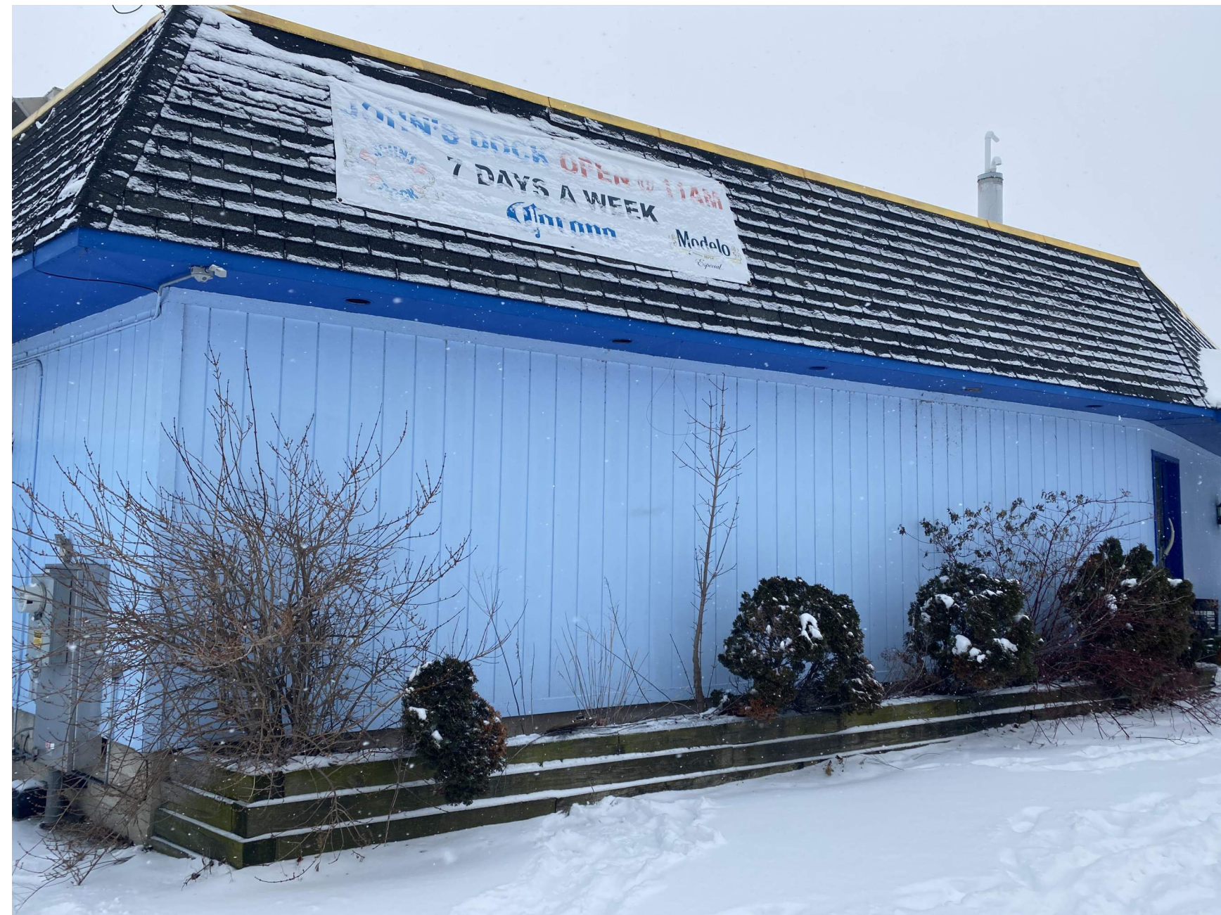
EXISTING BUILDING FRONT (NORTH) FACE
