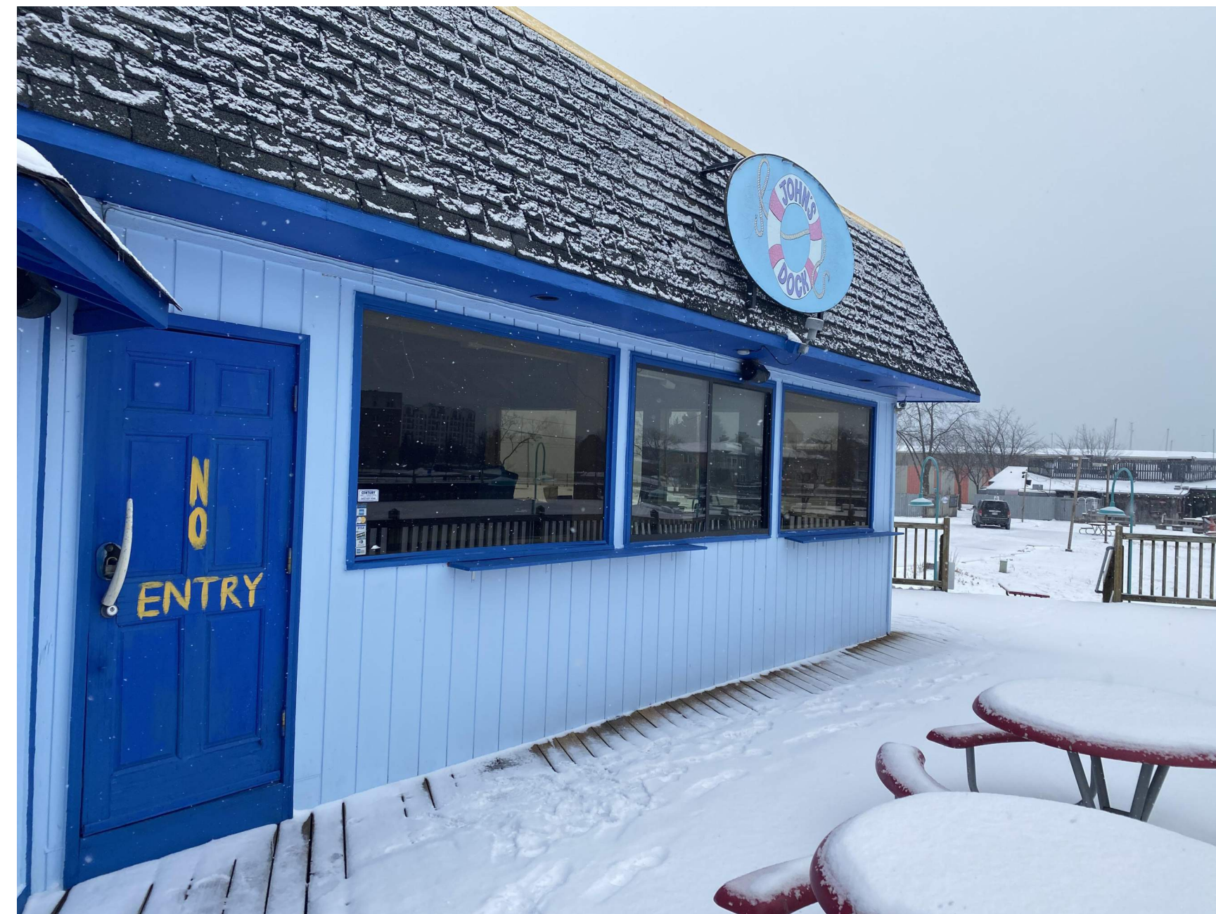
EXISTING BUILDING REAR (SOUTH) FACE
