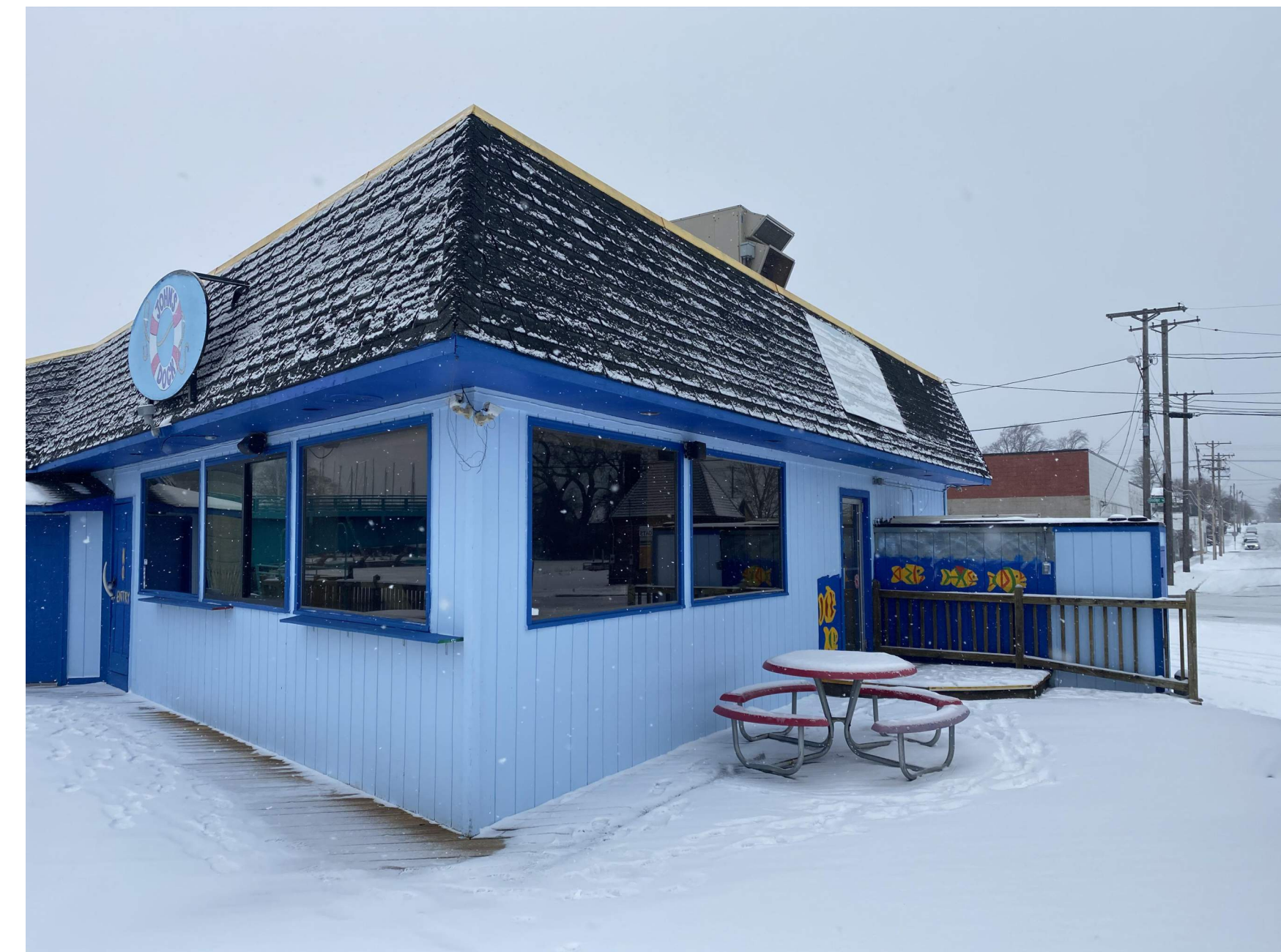
EXISTING BUILDING SE CORNER
