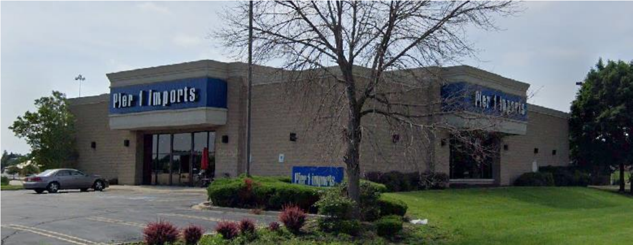
Existing building west and north façades.
