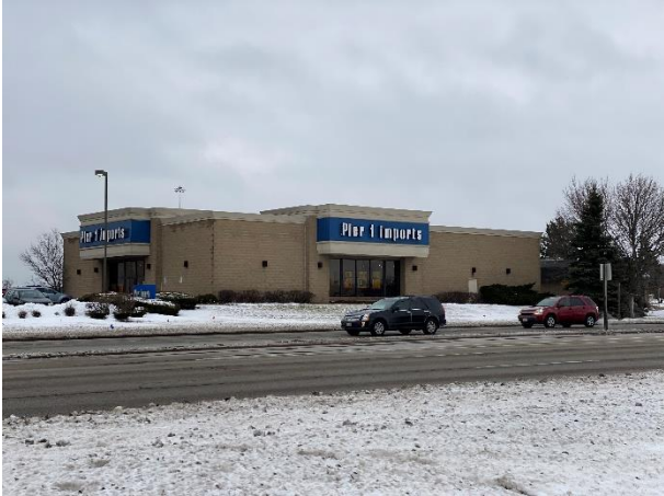
Looking southeast at existing building from S. Green Bay Road
