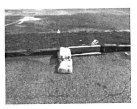
containment barriers will be installed before storm drain openings to capture residual water and color that could travel to the already installed visqueen media barriers. Leftover residual water that does not evaporate will be removed along with any remaining color.
