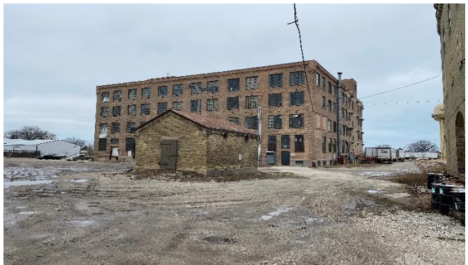
Looking northeast at 2234 Northwestern Avenue
