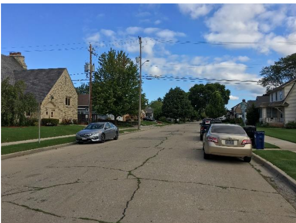
Looking north from subject property along Lawn Avenue
