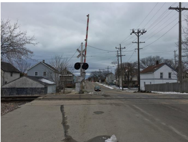
Looking east on High Street from access drive
