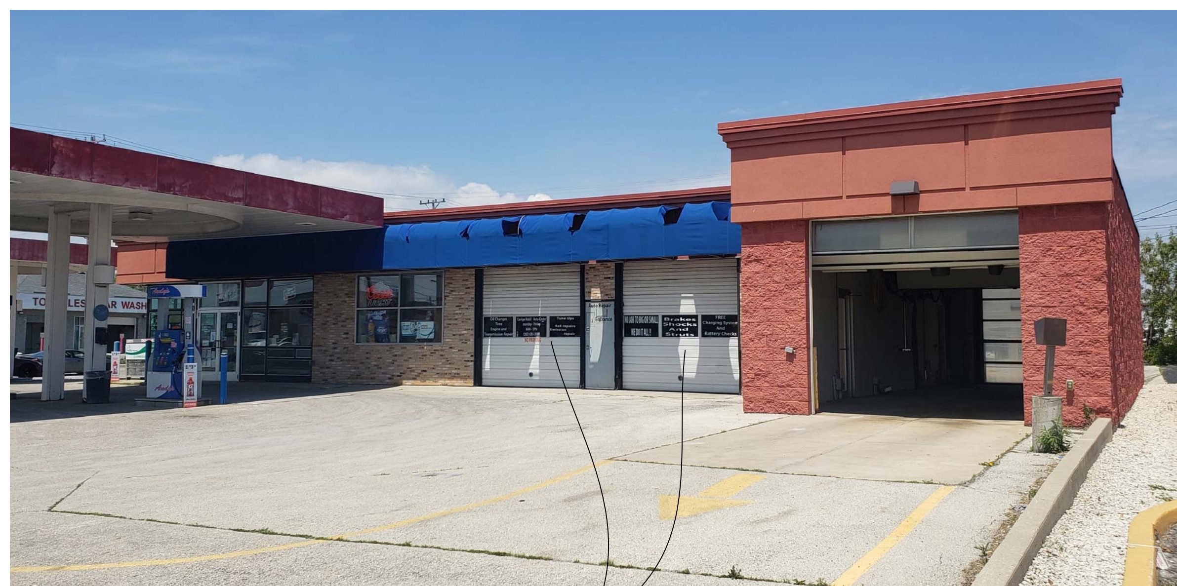
THE STOREFRONT GLAZING TO GO WHERE THE EXISTING OVERHEAD DOORS ARE LOCATED
