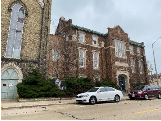
Looking East at subject property
