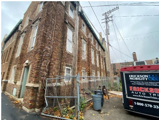
Looking North at rear of building
