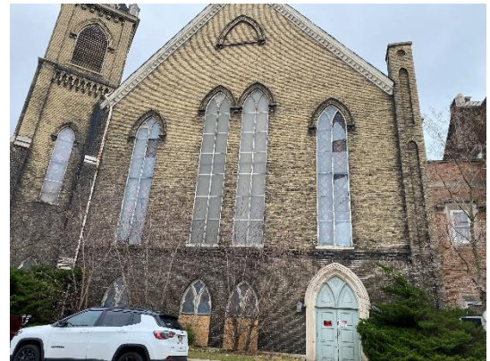
Looking East at Church structure
