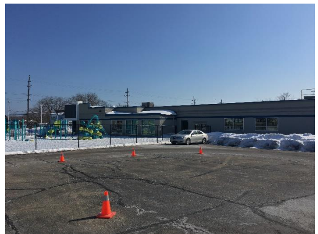
Looking towards north façade where proposed addition would occur
