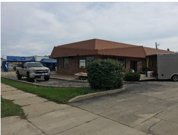
Looking at north façade of subject property
