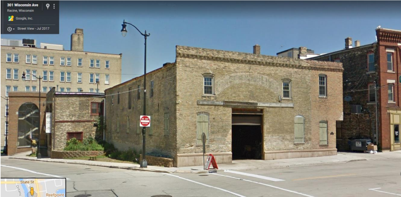
Looking to northeast
