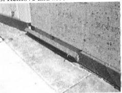
c. Install stainless steel strap anchors (two per base trim). Use existing slot in top of base. Saw new slot where none exists.
