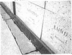
d. Replace pins in base trim where missing and drill dowel holes in newly cut edge of bottom shutters
