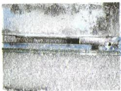
c. Replace cracked vertical trim with removed base trim where noted
