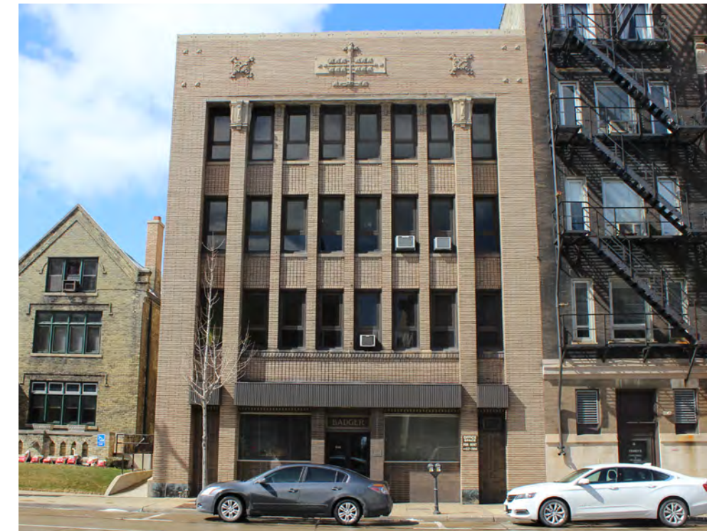
Badger Building - 610 Main Street
