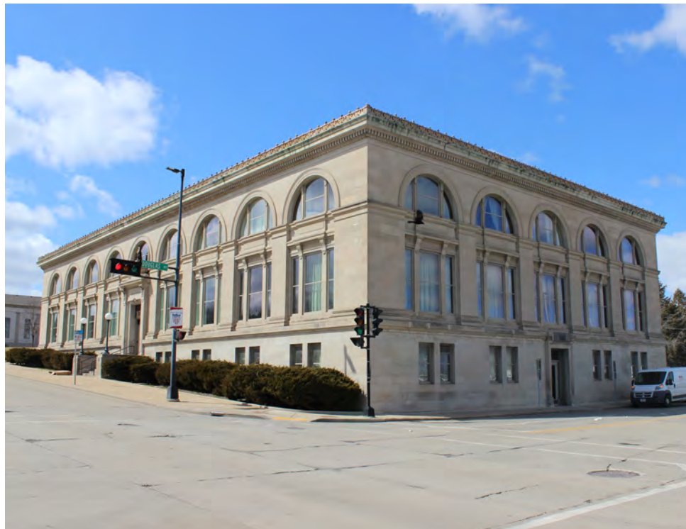
Jl Case Administration Building - 700 State Street
