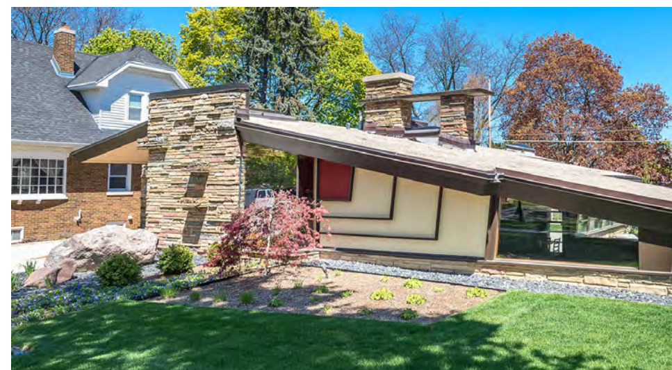
(Top) Demolition of Racine's Venetian Theater, (Middle) Downtown Racine circa 1960, (Bottom) Mid-Century Home at 1001 Russet Street.
