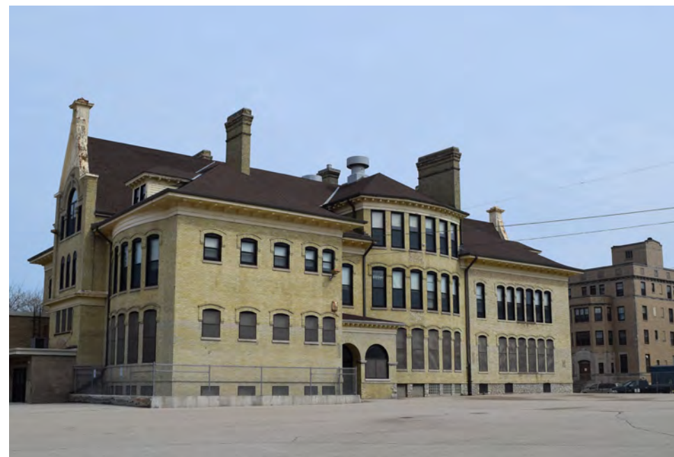
Closed Winslow Elementary School 1325 Park Avenue.
