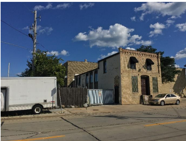
Looking at the north side of the property
