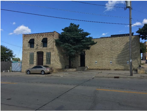
Looking at west side of subject property from Erie Street
