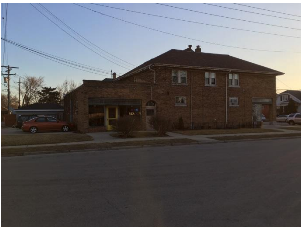
Looking (south) at subject property from Romaine avenue
