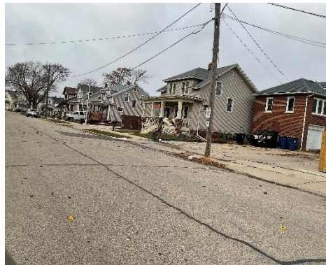
Looking Northwest down 20 th Street
