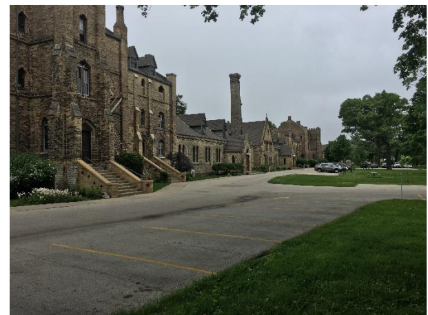
Looking northerly from the southeastern corner of the property
