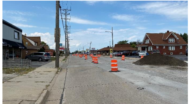
Looking north from subject property
