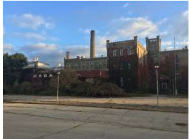
Looking north at 2100 Northwestern from front parking area
