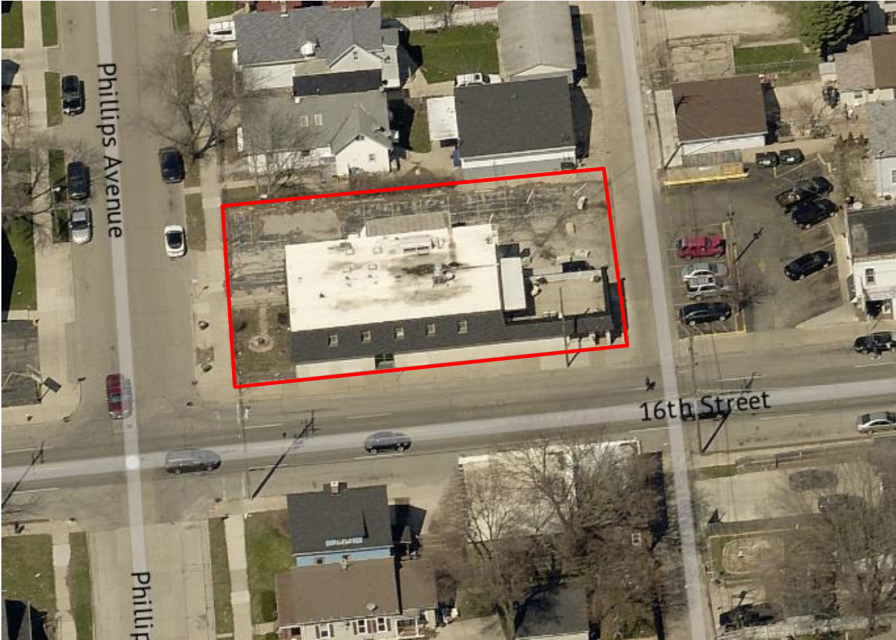
Birdseye view of the property, indicated in red, tenant space shown as purple (image from City Pictometry).
