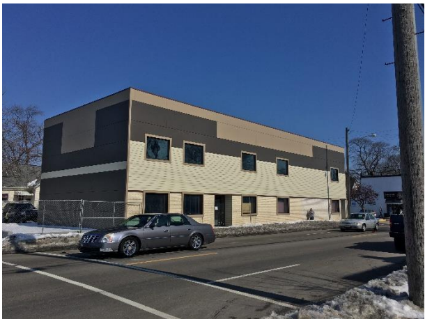
Looking northeast at the front of the building in existing conditions
