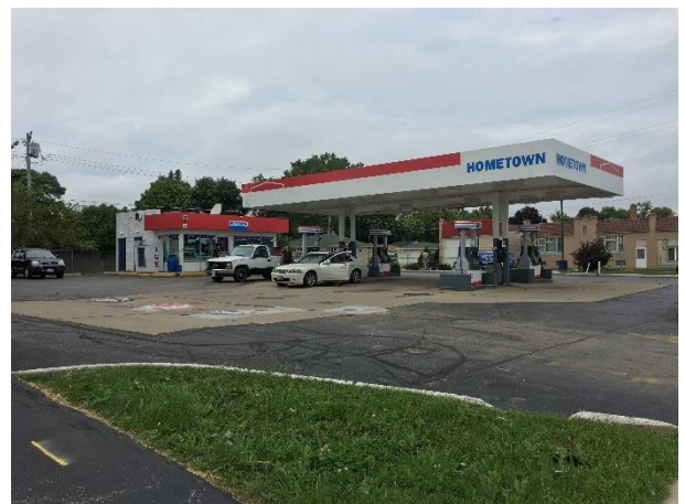
Looking northwest at the subject property
