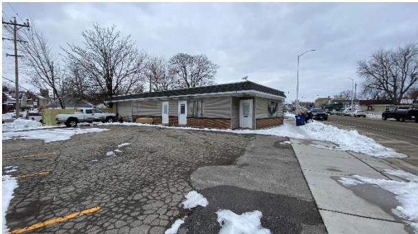
Looking north at building from Douglas Avenue
