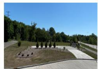
Lift Station #2 Storage
