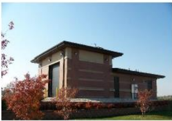
North Side Storage
