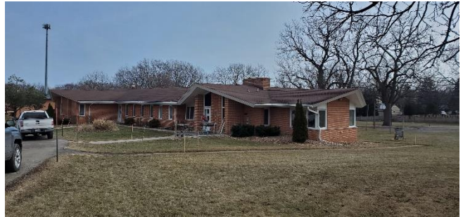
Looking east at subject property
