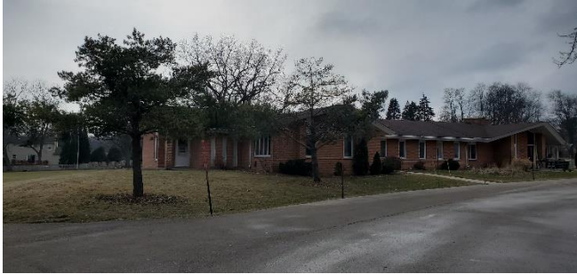
Looking south at subject Building
