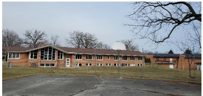
Looking north at the rear of subject building
