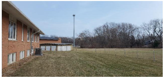
Looking west from subject building
