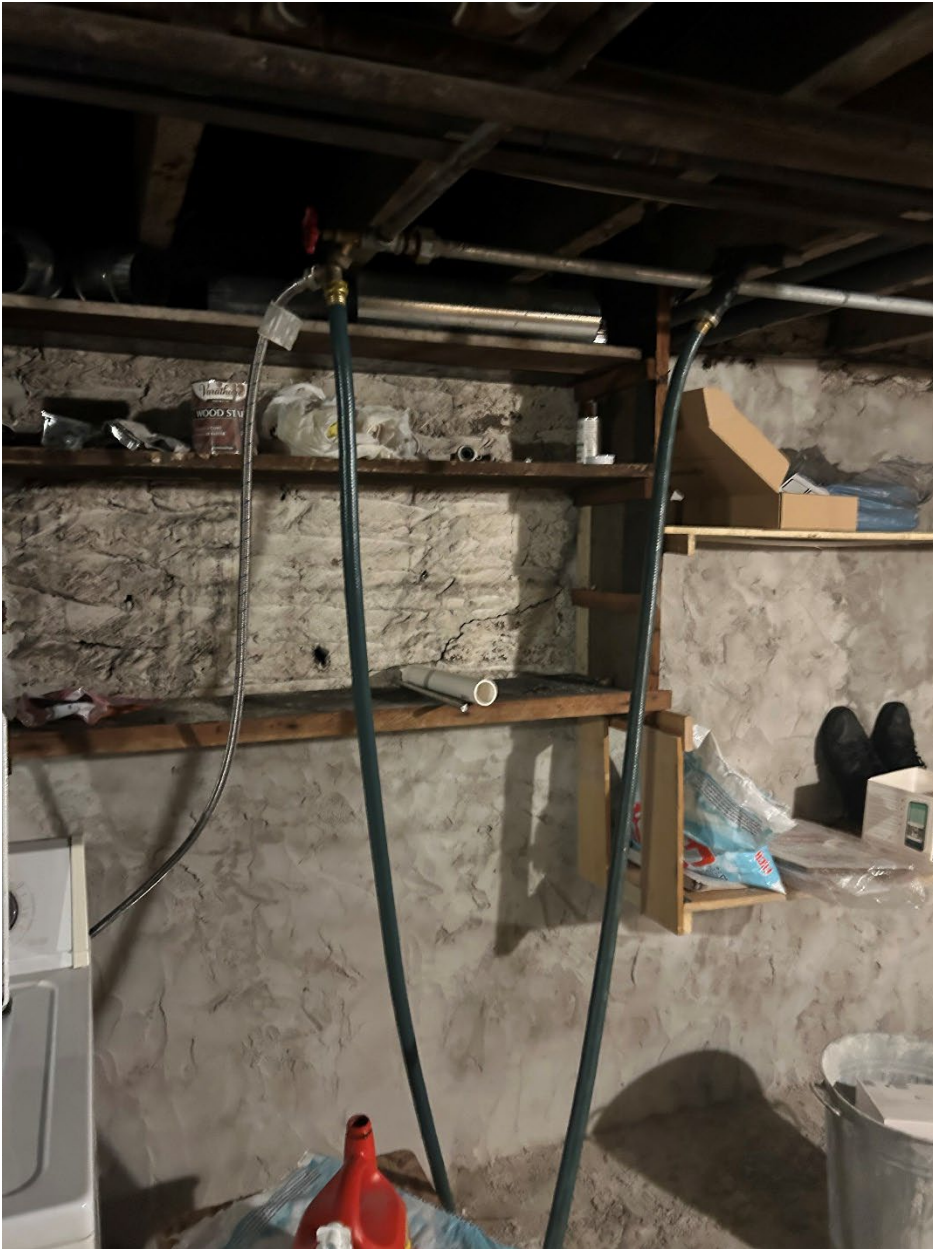
Basement – Photo shows that failed occupancy inspection for plumbing violation is still in violation
