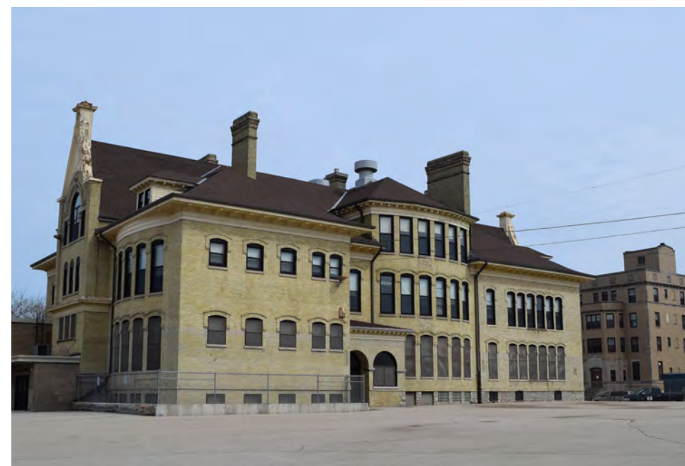
Closed Winslow Elementary School 1325 Park Avenue.
