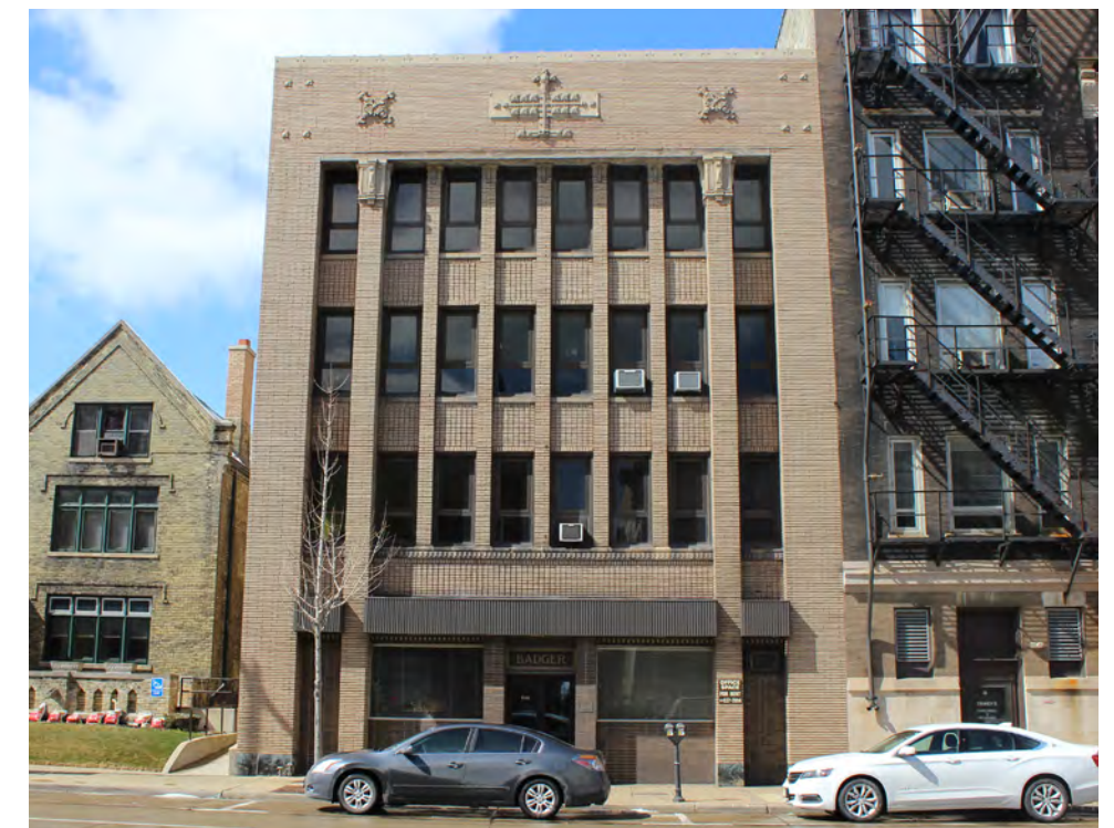
Badger Building - 610 Main Street
