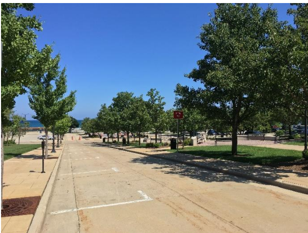
Looking east along Sam Johnson Parkway
