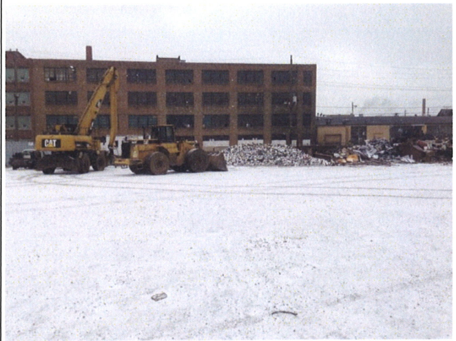
Photo No: 4 Picture Direction: N
