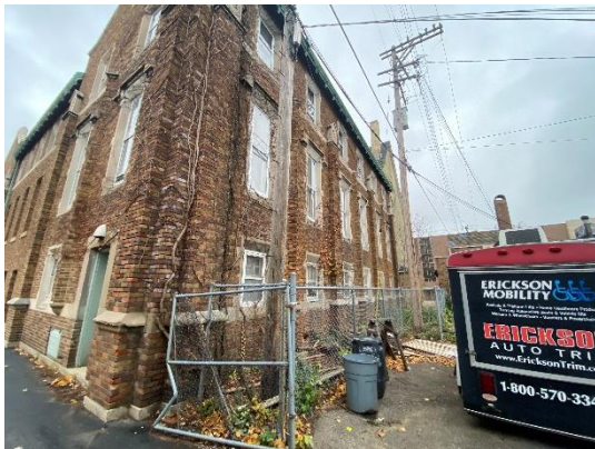
Looking North at rear of building
