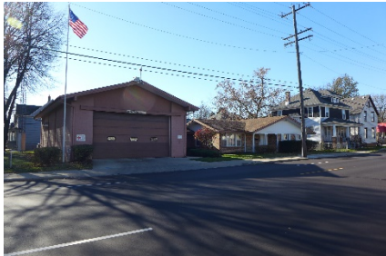
Front view of Fire Station 6
