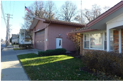
Fire Station 6 - Exterior
