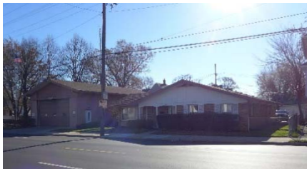
Front view of Fire Station 6
