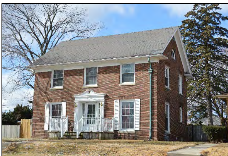
Nels H. and Elsie Peterson House, (1929) 1728 Carlisle Avenue
