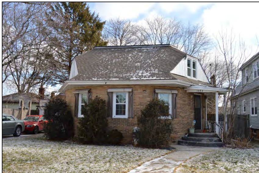
Elmer and Viola Hochgurtel House (1947), 1843 Blake Avenue, designed by Anton Kratochvil
